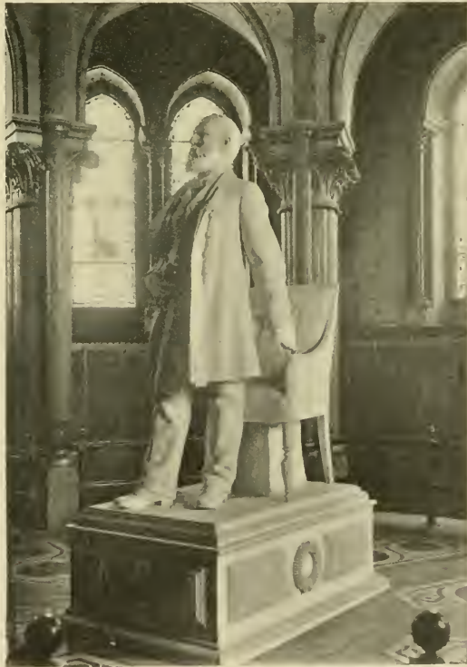
INTERIOR OF MONUMENT.
