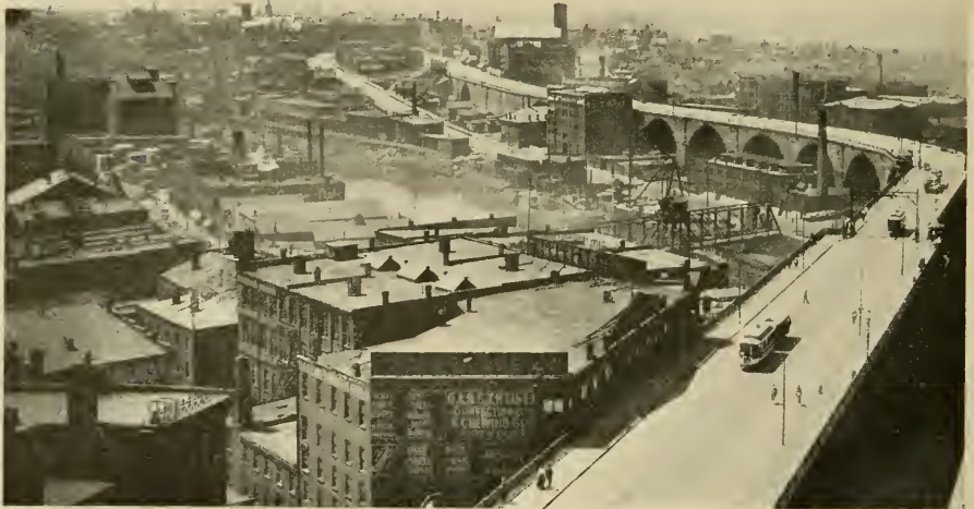
THE SUPERIOR STREET VIADUCT.
